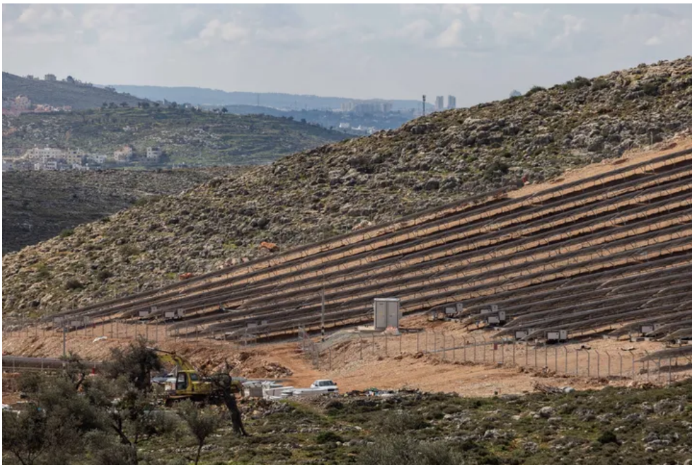
Solar panels near Deir Abu Mashal. Credit: Hadas Parush
